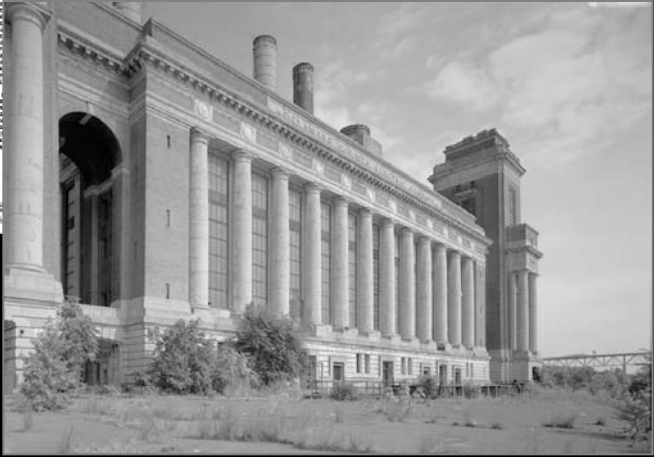
Chester Electrical Power Station, Chester, PA
