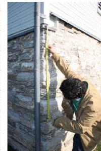
Measuring to the datum, Secondary House
